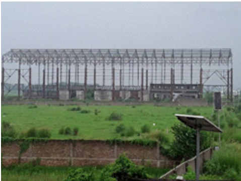
Figure 3.2: Incomplete Raw materials Processing Facility
