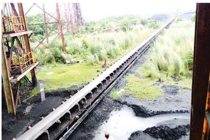
Fig. No. 3.2: Conveyor belt and stack yard of DPL
