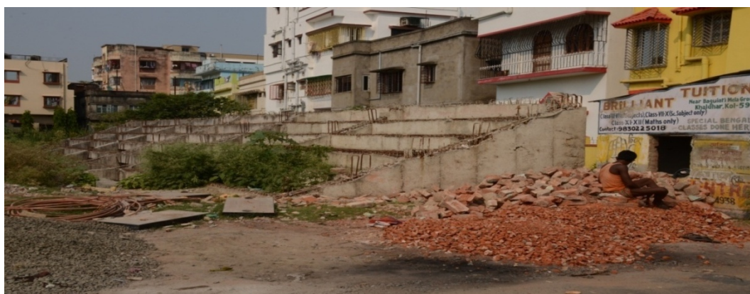
Incomplete works of stadium at Narayantala as on 24 March 2015
